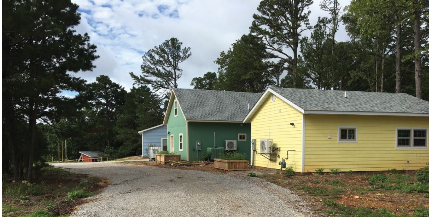
Since breaking ground on ECHO Village in June 2018, a total of eight small homes have been completed with another two under construction targeted for completion in August 2019.
